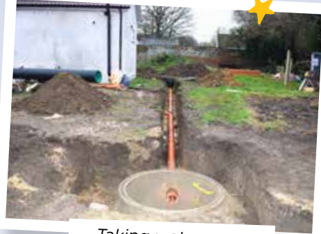
Taking water away from the building.
