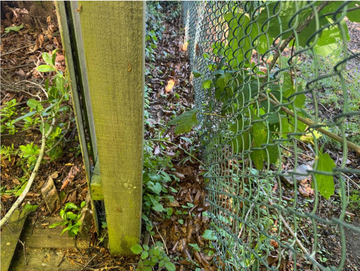
Photo 7. Looking down between chain link fence and panel fence along northern boundary of site.
