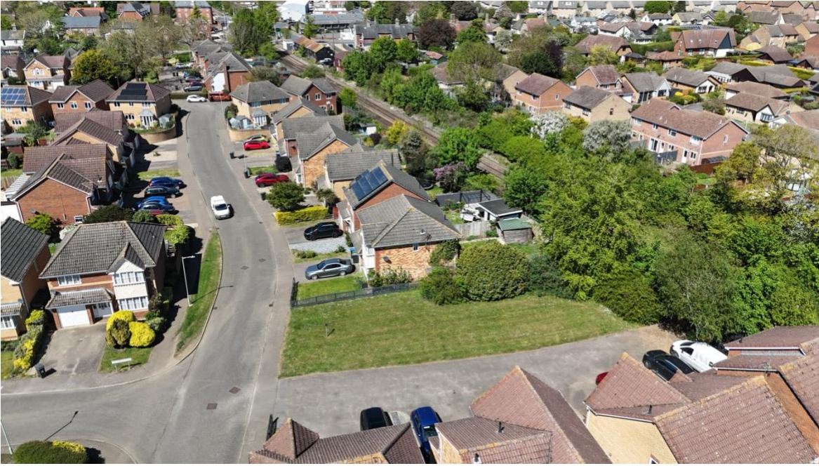
Photo 1. Aerial view of site. Looking northwest.
