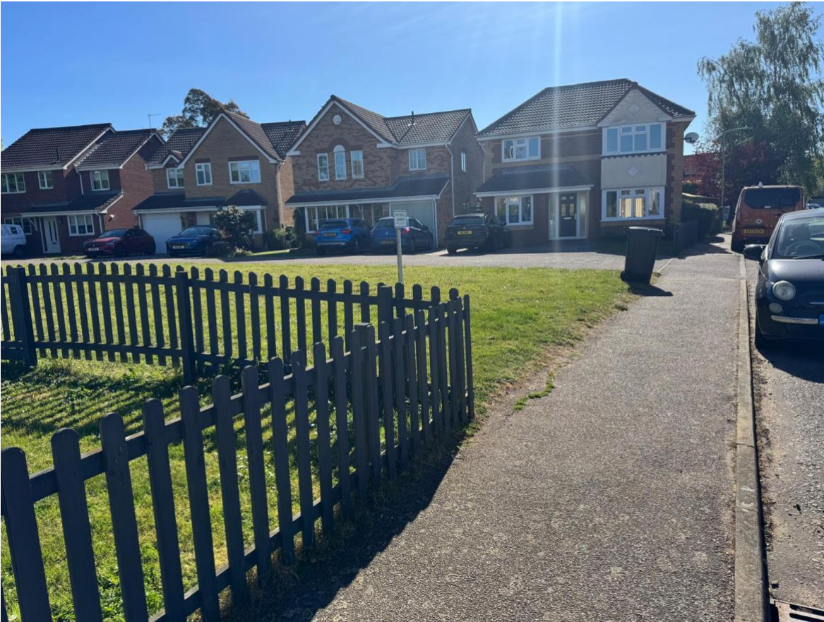
Photo 5. Taken from tarmac pathway along Crown Mill. Shows picket fencing. Looking east.
